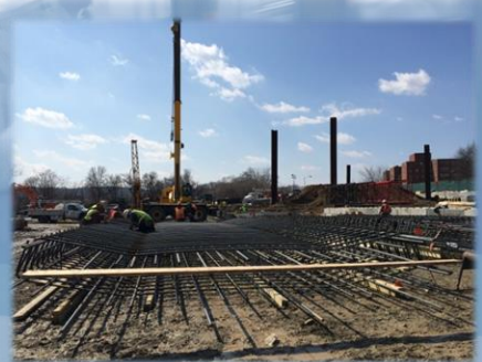
Primary Panel Rebar Cage Fabrication
