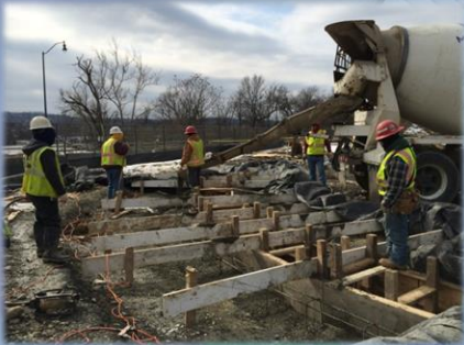
Placing Concrete for Guide Walls
