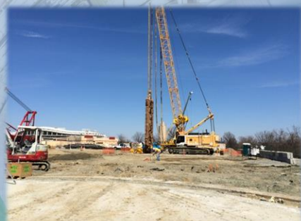
Hydromill for Slurry Wall Panel Excavation
