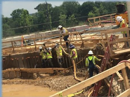
Preparing Top of Slurry Wall for Capping Beam Installation
