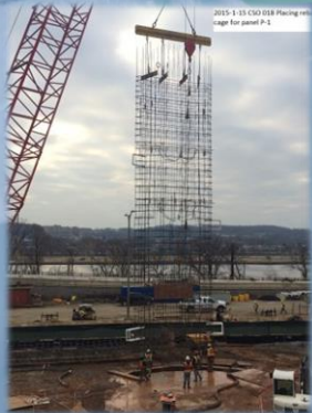
Placing Rebar Cage for Slurry Wall Panel
