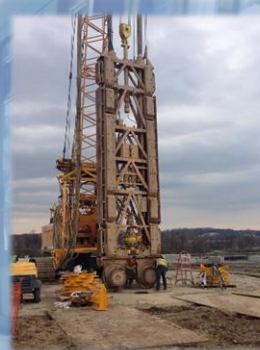
Hydromill for Slurry Wall Panel Excavation
